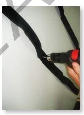
Step 2: Open the wall brackets and place them on the desired area. Then screw them tightly using 2 screws in each one.
